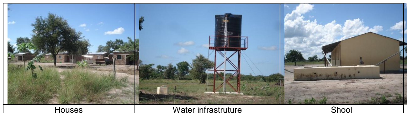
Figure 14: Construction of habitations and infrastructures in the resettlement area (18 Km from Nova Mambone village)
